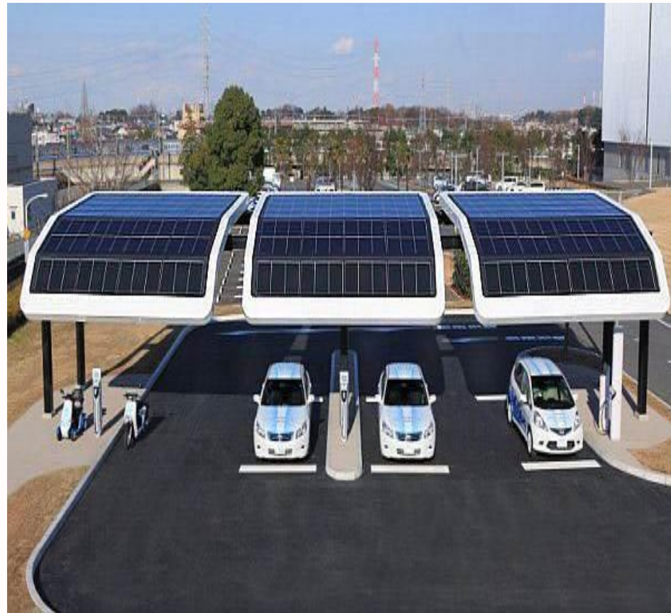
光伏充电系统 Photovoltaic Charging System
