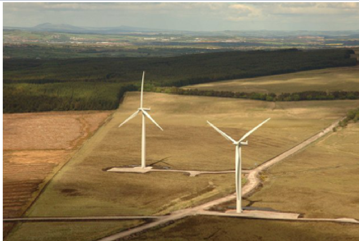
Two of the wind turbines at the Black Law Wind Farm in Scotland
