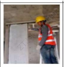
⑩加固管卡射钉与 结构锚固
